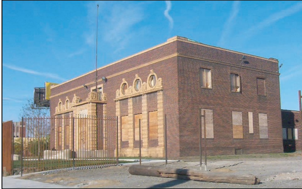
Façade and East Elevation
