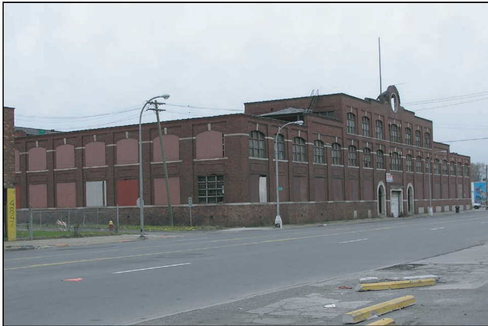
C-9. Roberts Brass Manufacturing Company Building, 5436 West Fort Street
