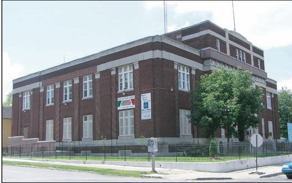
Façade and East Elevation
