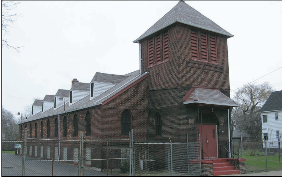
Façade and North Elevation
