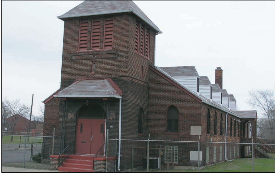
Façade and South Elevation
