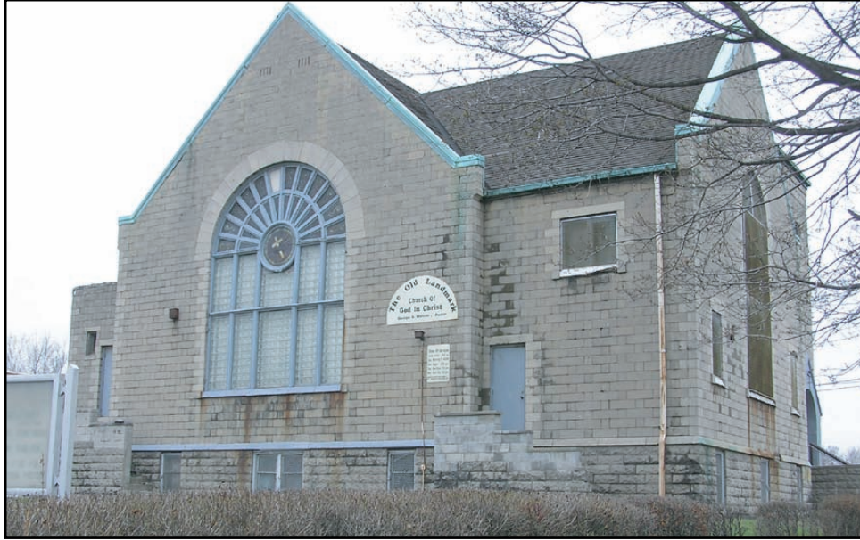
South and East Elevations
