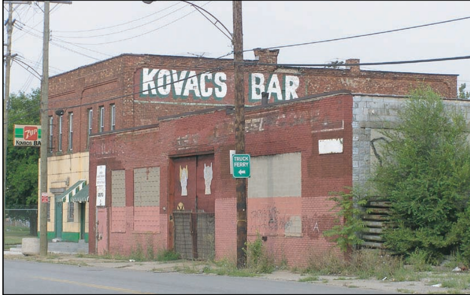
Streetscape of Building From West Jefferson Avenue, View Northwest
