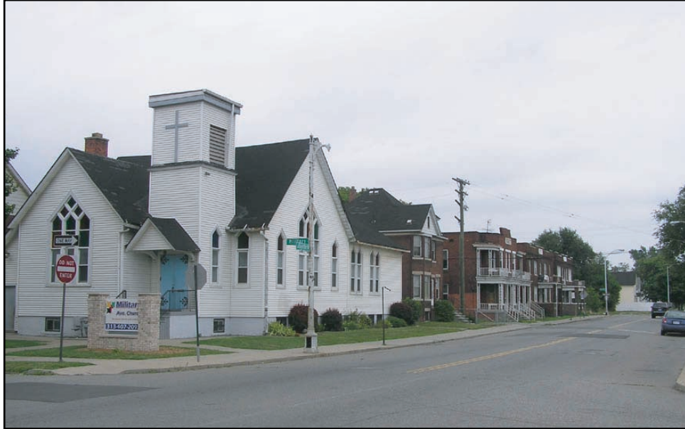
Streetscape along West Lafayette Boulevard, View Northeast
